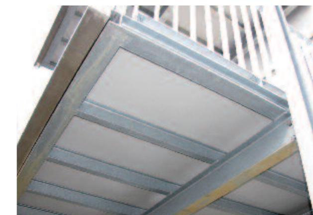
substructure/bottom view of terrace floor
